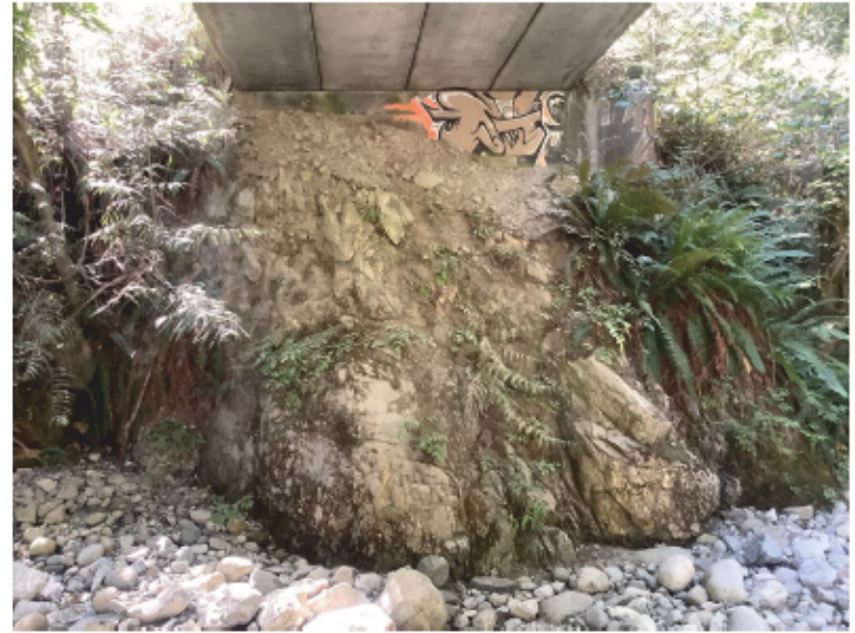
Left Bank Abutment when facing downstream
