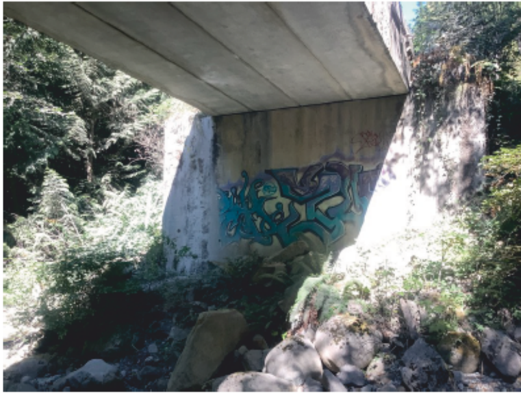
Right Bank Abutment when facing downstream
